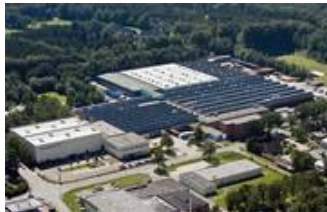
The Grundfos pump factory in Wahlstedt has been equipped with EnwaMatic® Technology.
